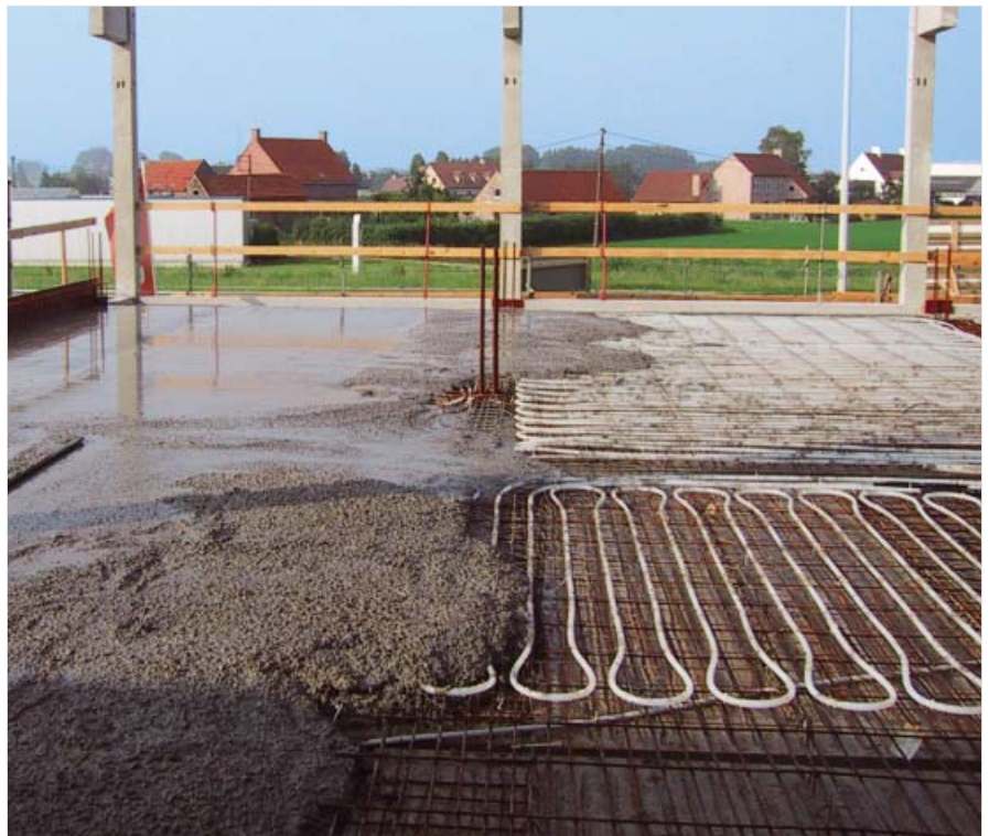
Fig. 11: Using a building component/concrete core – creating an intermediate layer with pipe system
