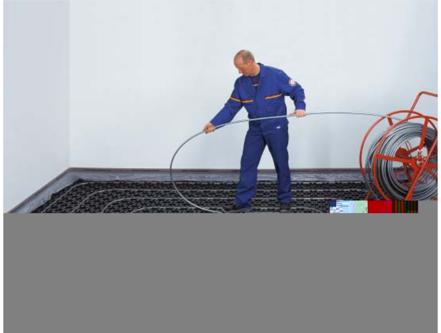
Fig. 10: Installing an underfloor heating/cooling system
